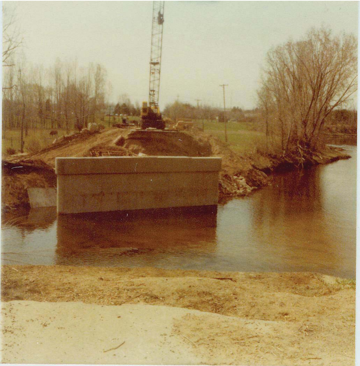
Chippewa River Bridge Construction
